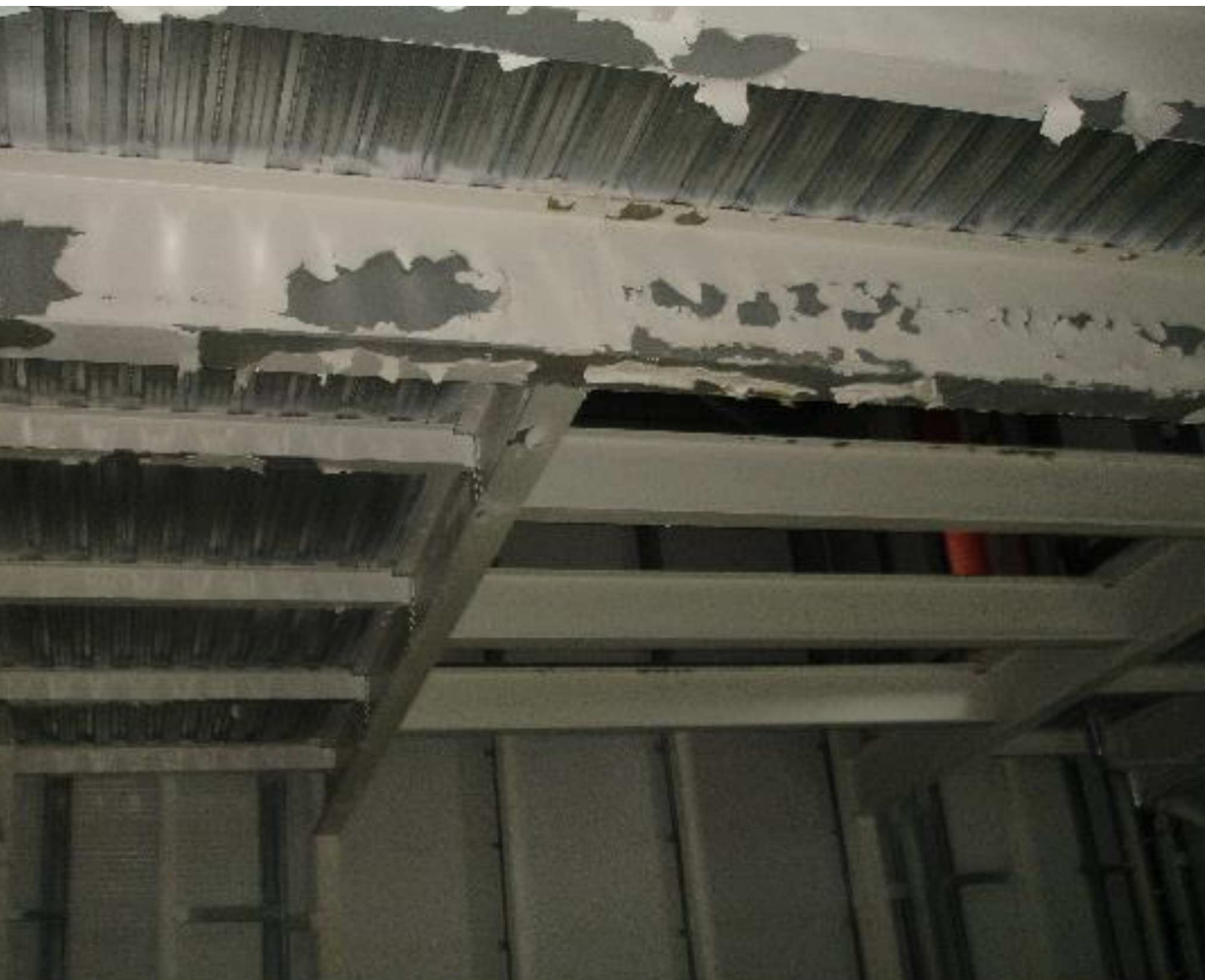
Defective paintwork on interior steel frame
